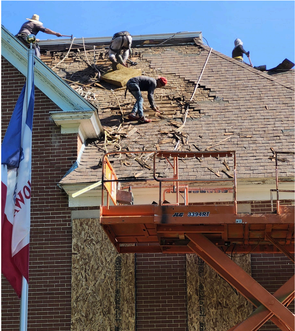
Ripping off the old layers of roofing materials. 25 June 2024. Over twenty workers stripped the entire roof and installed the OSB board in one day.
