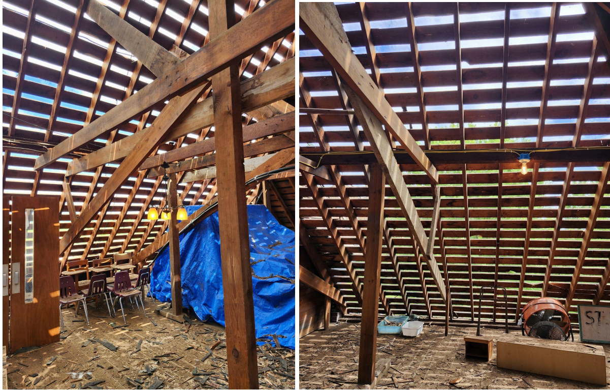
Roof Structures After Three Layers Were Removed. 25 June 2024
