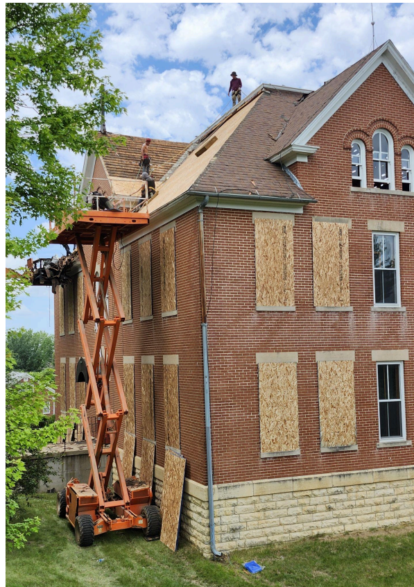
Installing the OSB plywood sheets.
