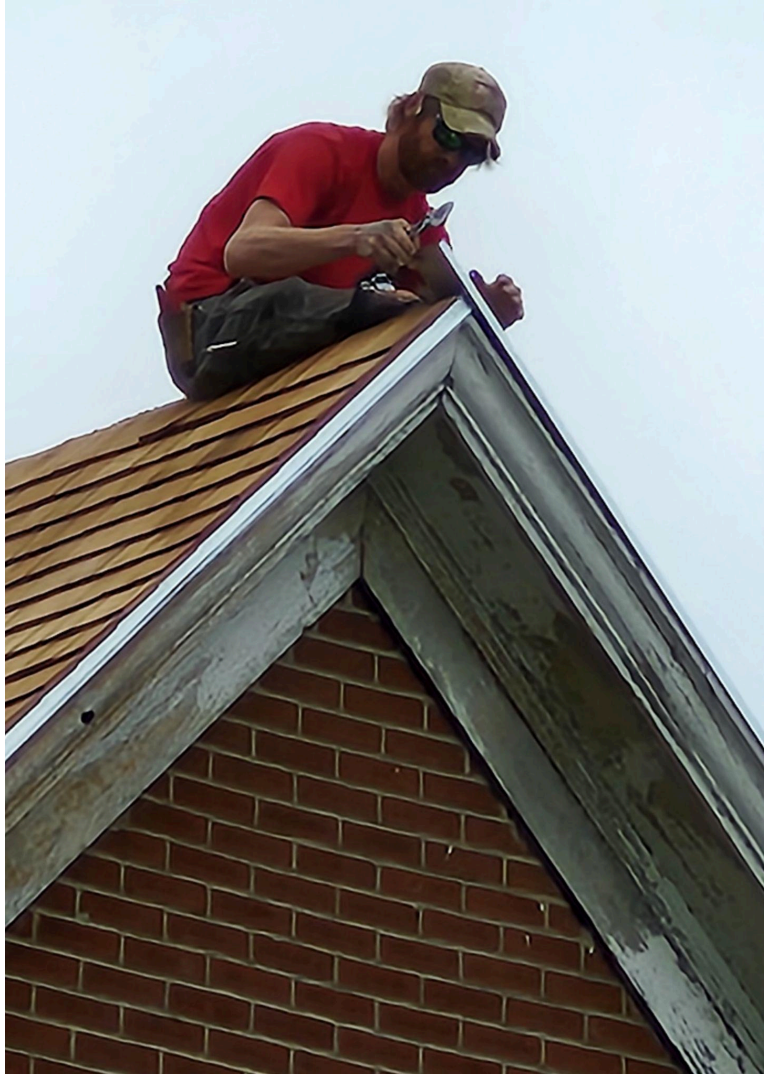
Placing water guard on North slope of East Gable of German American Museum, August 8, 2024.
