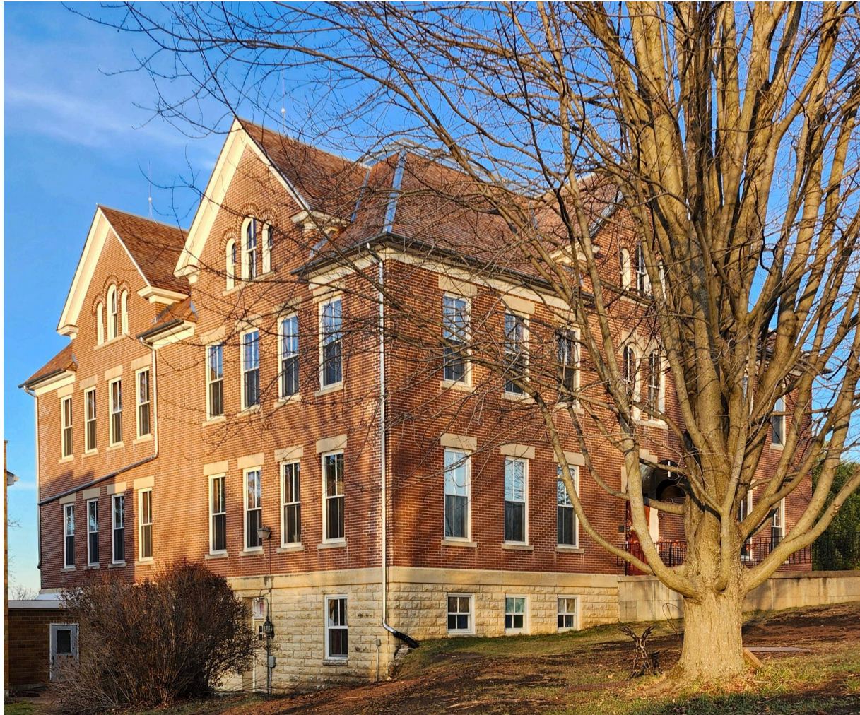
Roof Rehabilitation Project Completed with red cedar wood shingles, galvanized ridge liners, new gutters and downspouts, two new rubber flat roofs, lightning rods with glass bulbs and newly painted soffits. November 9, 2024.
