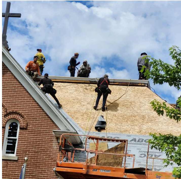
New OSB board going on the roof.
